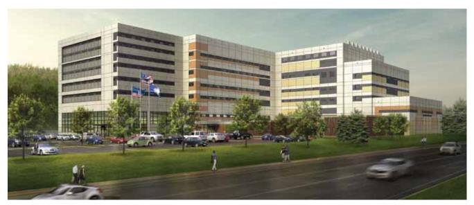
A total-precast concrete structural solution was selected for the \$134.6-million, 1,032-bed Richmond Justice Center, which is now being constructed. It features quad cell units, double tees, columns, beams and exterior load-bearing architectural insulated sandwich wall panels. The panels are being cast with the use of form liners that hold thin brick which are embedded in the building façade to create a contextual and rhythmic design.
